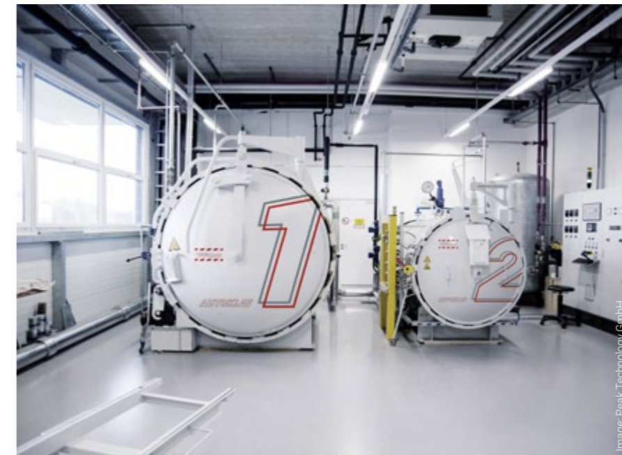
Wound and laminated parts are cured under pressure in the autoclave.
